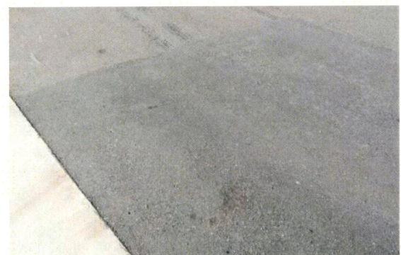
T-Lock repair with the GlasGrid System
