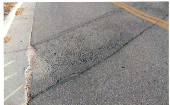
T-Lock repair without the GlasGrid System
