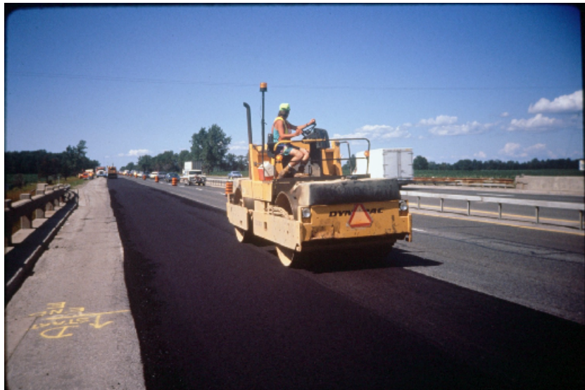
Figure 20. Compaction of the longitudinal joint from the hot side
