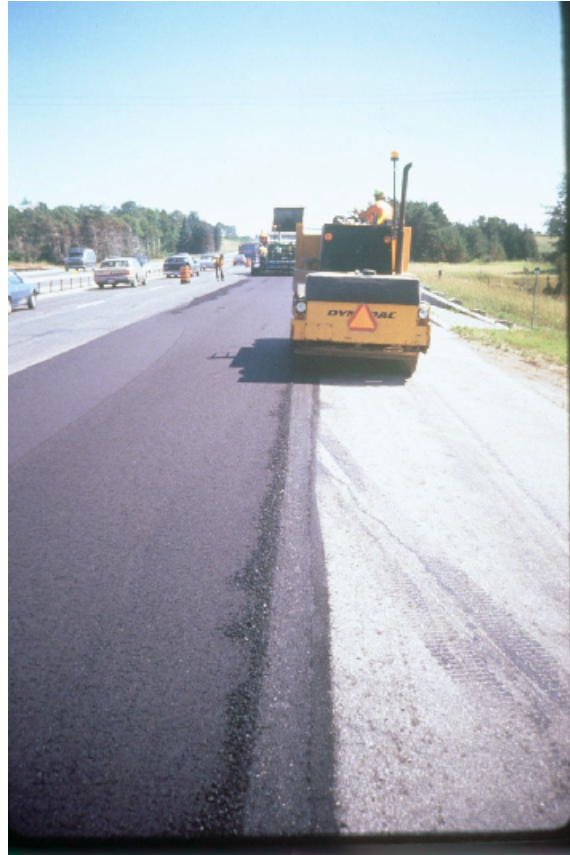
Figure 17. Compaction of the longitudinal joint from the cold side
