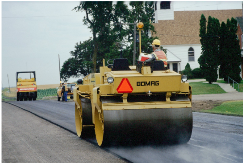
Figure 10. Edge of the roller drum extended over the unsupported edge of pavement
