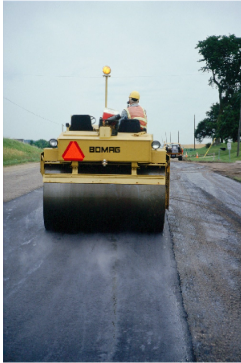
Figure 6. Edge of the roller drum inside the unsupported edge of pavement
