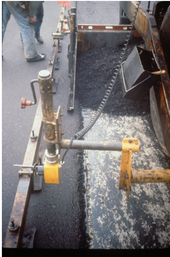
Figure 15. Proper amount of overlap of mix from lane 2 over lane 1
