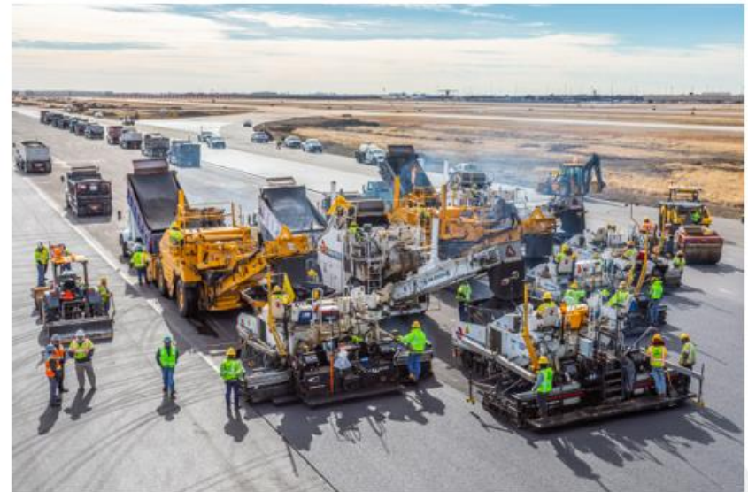
Figure 9.22 Echelon Paving with Four Paving Trains on a Runway at DFW Airport
