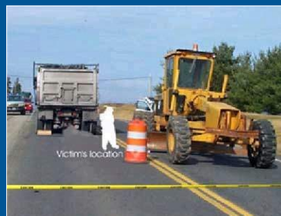
Figure in white shows where the worker was standing when he was run over. The driver did not see the victim.
