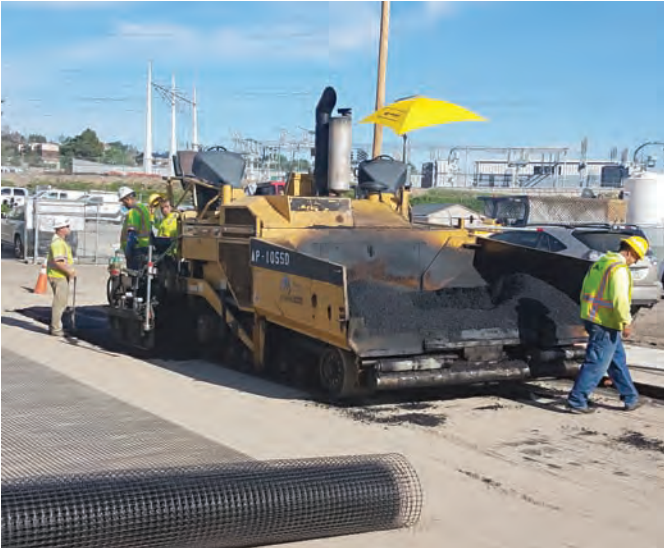
Full reconstruct in Phase 2 using geogrid
