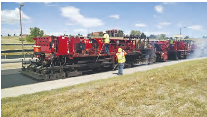
Hot In-Place Repaving in Thornton
