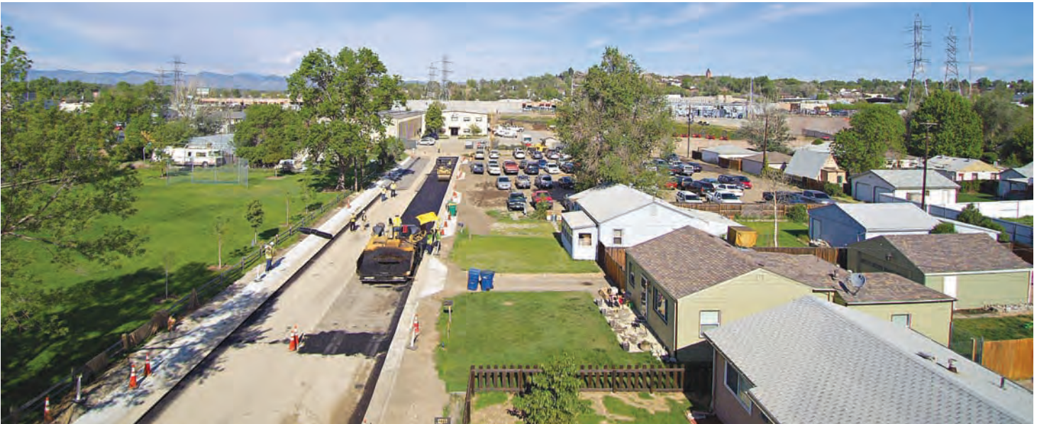
Full reconstruct in Phase 2 using geogrid
