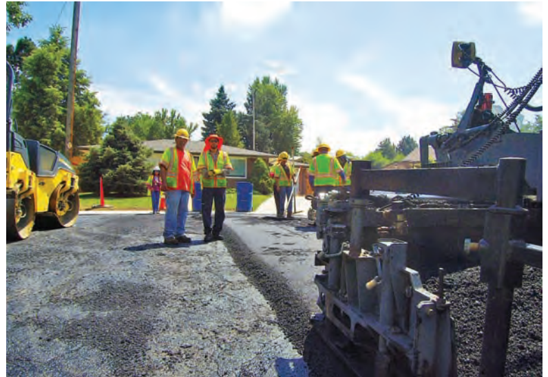
Mill & Overlay in Phase 3 (2017)
