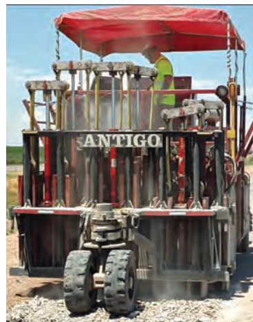
Rubblization process US Highway 85, Weld County
