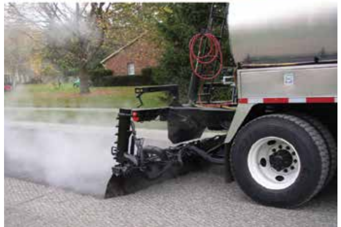
Figure 5-2 a and b. Uniform Tack Coat Spray Application
