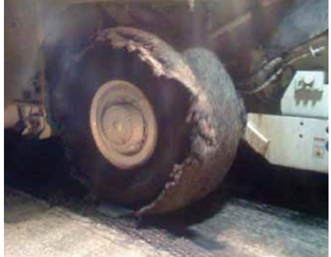
Figure 4-3. Tack Coat and Debris Picked Up by Construction Traffic From a Dirty Milled/Tacked Surface
