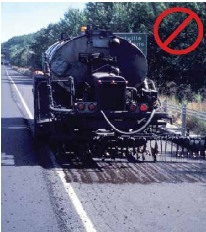
Figure 5-5. Non-Uniform Tack Coat Spray Application Due to Improper Nozzle Setting
