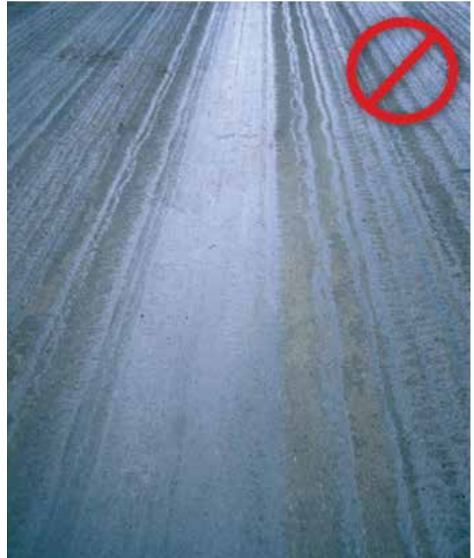
Figure 5-5. Non-Uniform Tack Coat Spray Application Due to Improper Nozzle Setting
