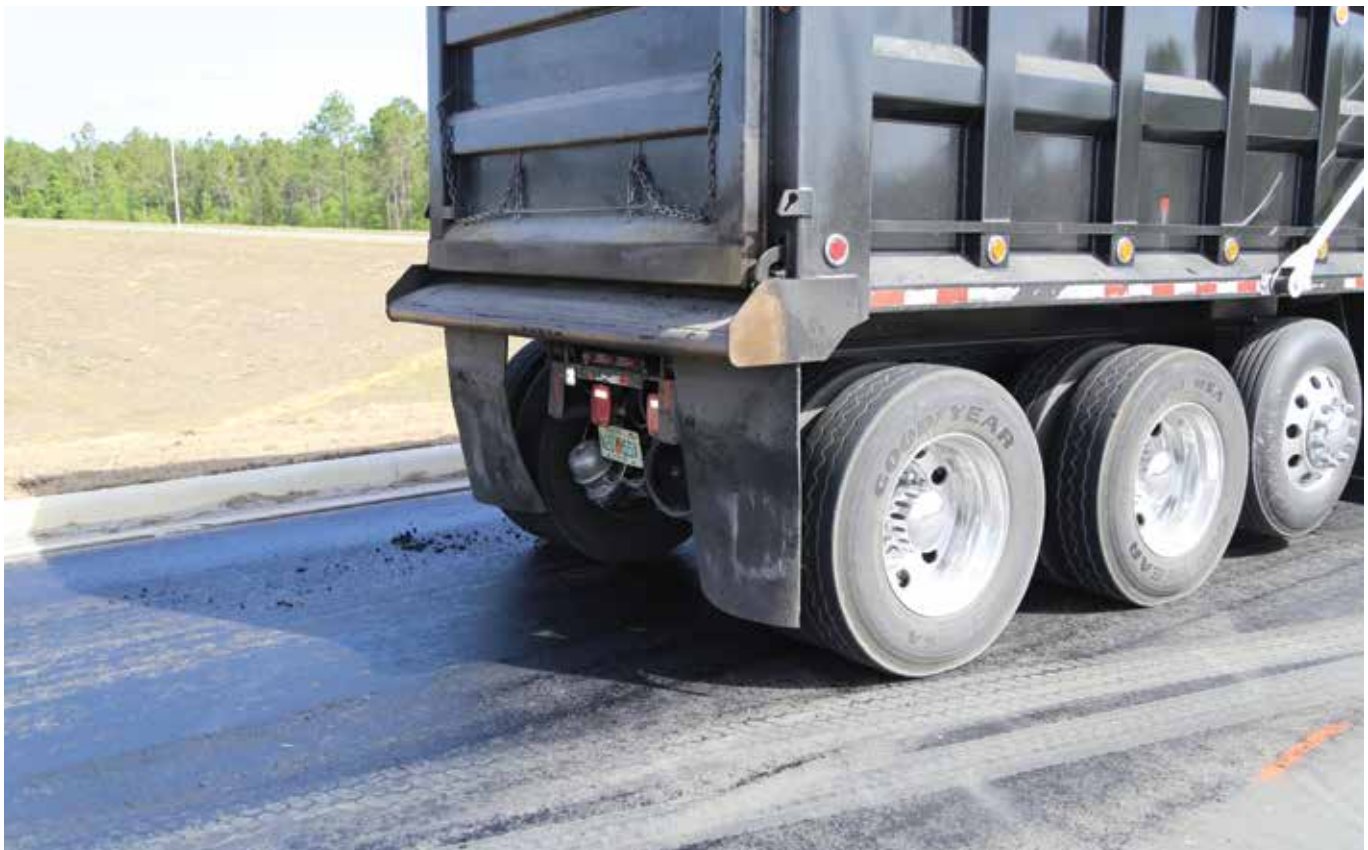
Figure 5-9. Pickup of Tack Coat Emulsion by Construction Traffic Should Be Avoided
