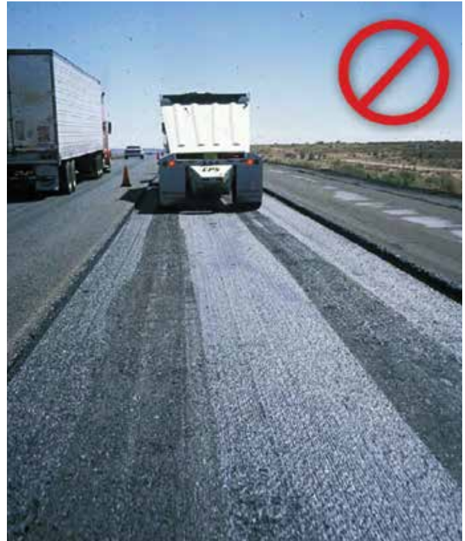
Figure 5-9. Pickup of Tack Coat Emulsion by Construction Traffic Should Be Avoided
