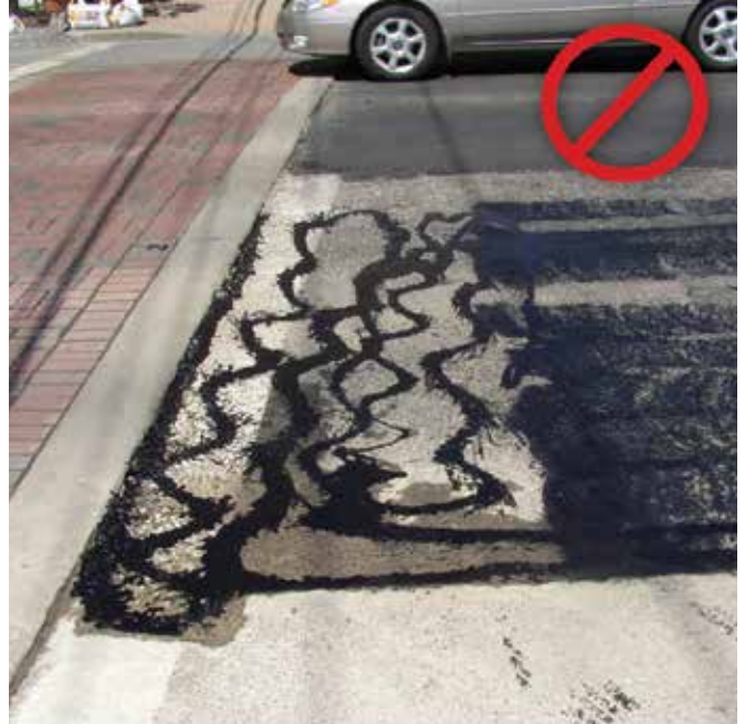
Figures 3-13 a and b. Improper Application of Tack Coat Using a Crack-Sealing Bucket
