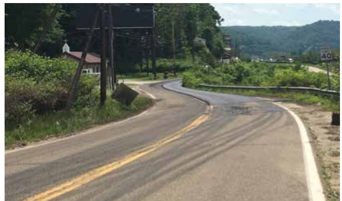
Figure 3. Tracked Tack Material (WVDOH)
