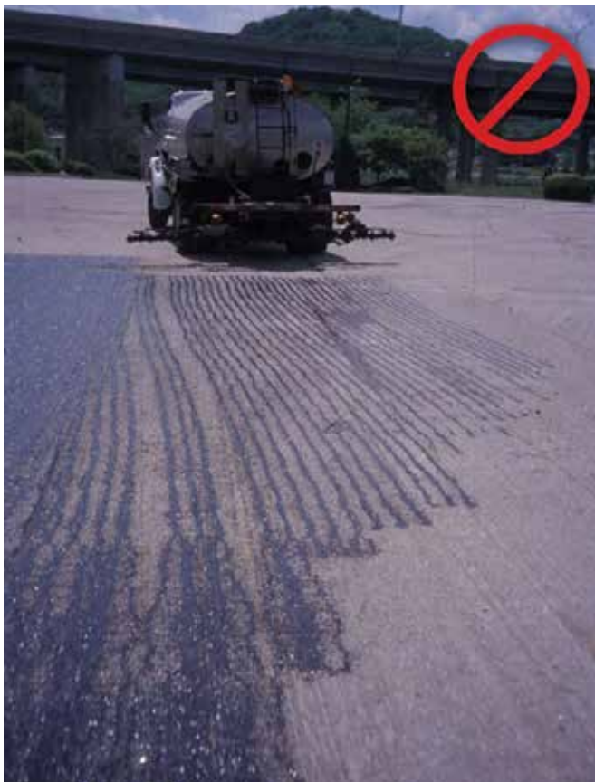
Figures 3-12 a and b. Tack coat Spray Applied With Plugged Nozzles Other Issues Can Also Result in a Similar Streaky Appearance
