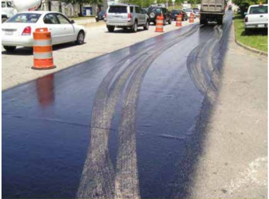
Figure 9. Tracking Due to Unclean Underlying Surface
