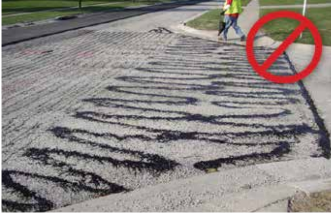
Figures 3-13 a and b. Improper Application of Tack Coat Using a Crack-Sealing Bucket
