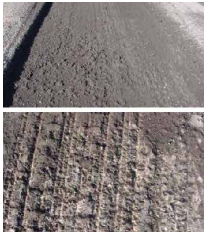
Figure 4-2. Clean Milled Surface
