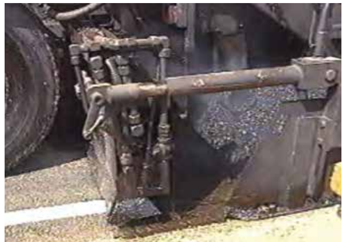
Figure 3-18. Tack Coat Application in Front of Auger Chamber Using Spray Paver
