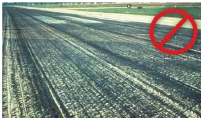
Figures 5-4 a and b. Non-Uniform Tack Coat Spray Application Due to Improper Nozzle Setting
