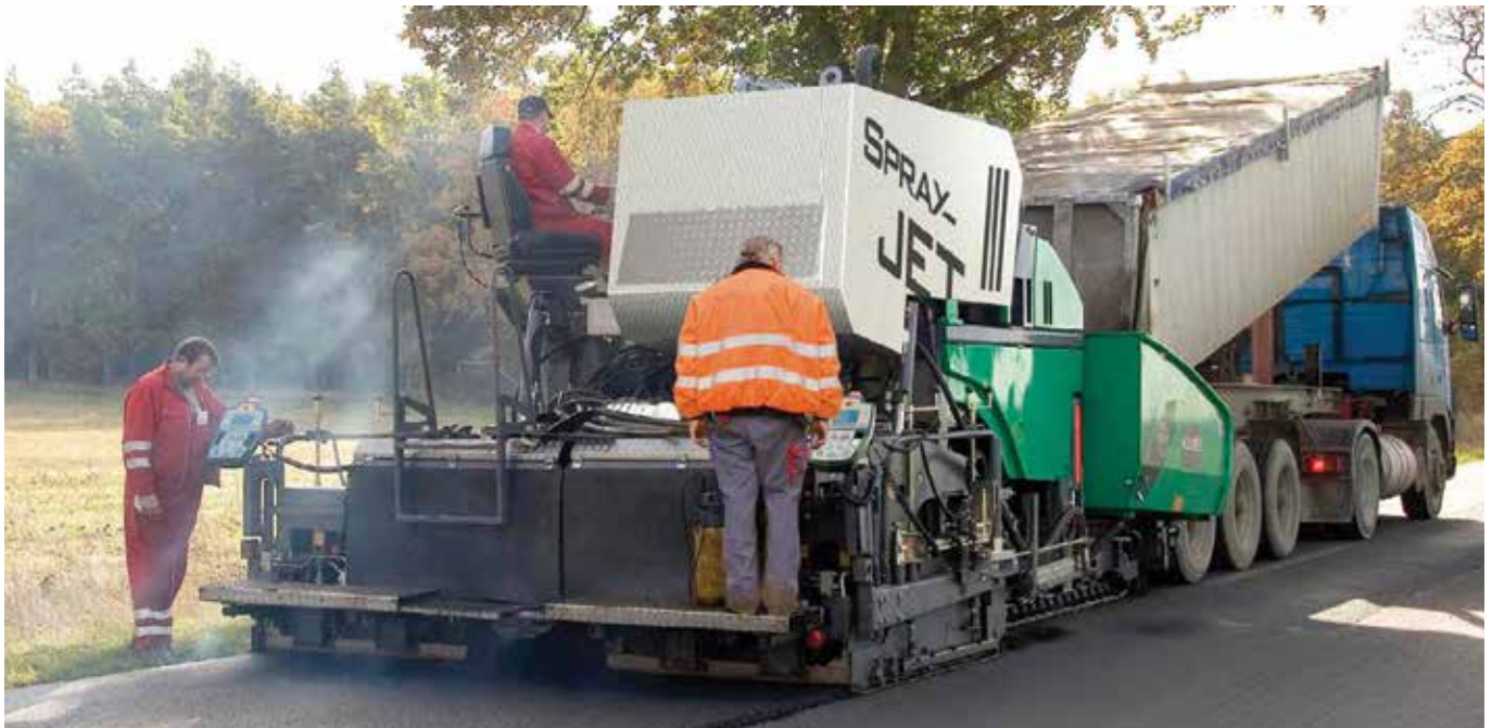
Figure 3-16. Asphalt Paver With Asphalt Emulsion Tank for Tack Coat
