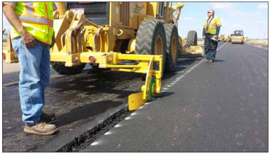
Pavement improvements at the Colorado Springs Airport, Summer 2014. Contractor: Schmidt Construction
