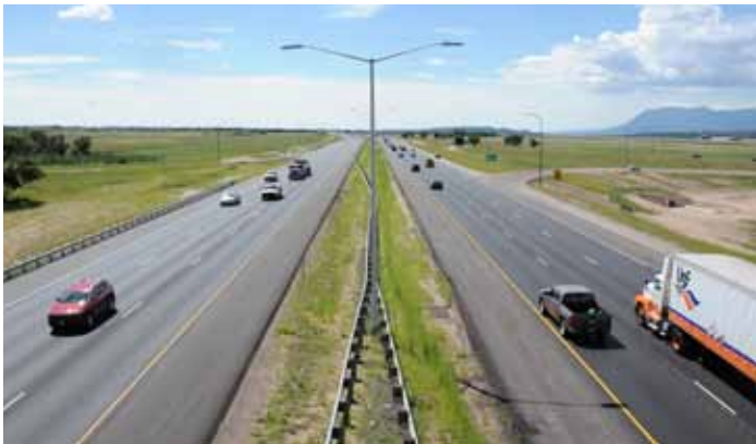
PROJECT: I-25, COLORADO SPRINGS TO MONUMENT CONTRACTOR: KIEWIT INFRASTRUCTURE OWNER/AGENCY: CDOT REGION 2
