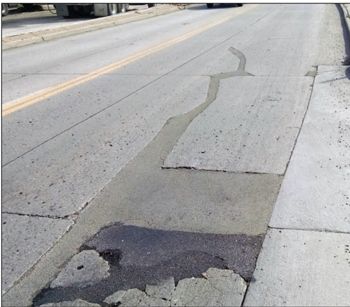
Existing concrete pavement to be removed along Mainstreet
