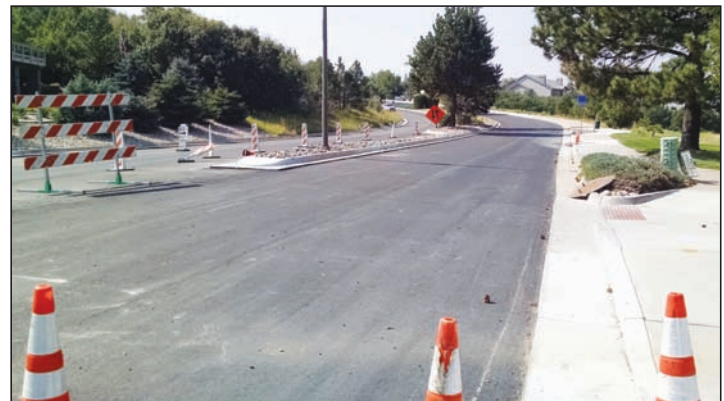
New asphalt pavement on Plum Creek Boulevard
