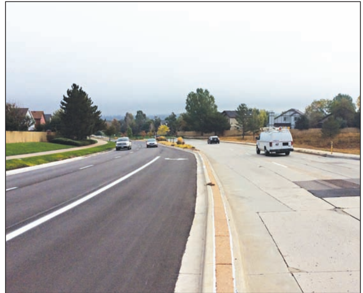
New asphalt construction along westbound lanes of Mainstreet
