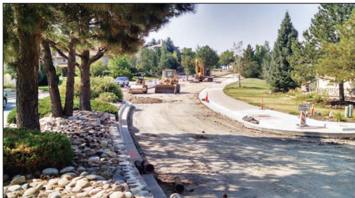
Removal of distressed concrete along Plum Creek Boulevard
