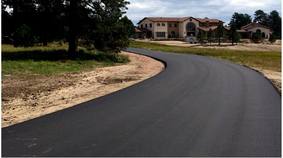
Asphalt pavement is a popular choice for residential driveways. Properly designed and constructed, it stays smooth, sound and attractive in appearance for many years. Flexibility allows the pavement to conform to minor settlements and still retain a continuous surface free of abrupt bumps. A well-designed, constructed and maintained driveway will give trouble-free service for up to 20 years and will add appeal and value to the property.
